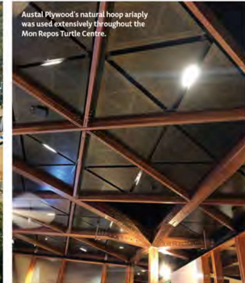
The use of sustainably sourced glue laminated timber was instrumental in meeting the project's 50-year design life requirement.
