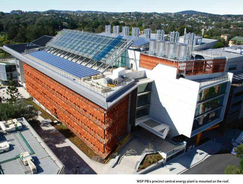
The pre-conditioned air it supplies is utilised as outside air provision for a multitude of air handlers, and to provide conditioning to the building's central atrium when suitable conditions prevail.
