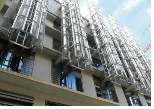
External ductwork risers contain various ventilation ducts that reticulate between plant rooms. They also provide shading for laboratories.
