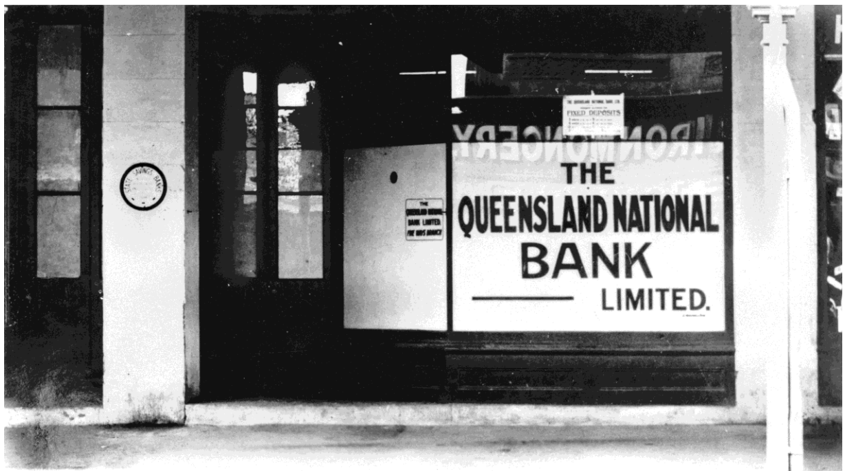
Temporary premises (Shop 15 or 17) of the Queensland National Bank, Logan Road, 1923–24 with signwriting for JR Blane's ironmongery (on the opposite side of Logan Road) reflected in the glass (SLQ).
