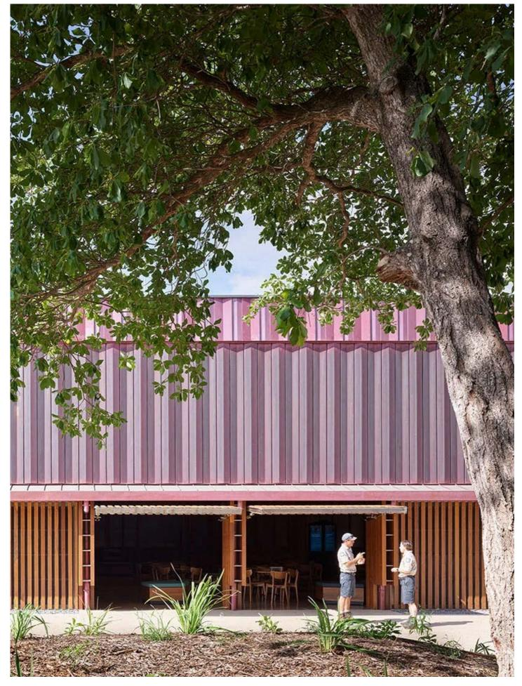
as well as responding sensitively to the site and forging a connection between visitors and nature, the project also embraces sustainable design by the use of a prefabricated structure of glulam timber. locally grown and manufactured, the structure was delivered and fully erected in 2 weeks, which saved valuable construction time and minimized transportation as timber members could be stacked in single lengths. erection occurred with a single mobile crane and less than a total of 2-4 riggers.
