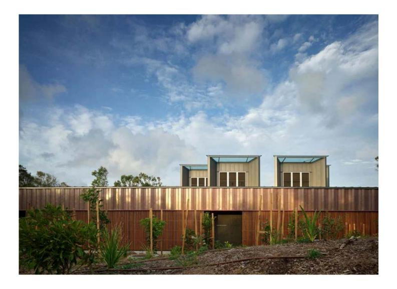
the use of timber also meant the project could fulfil the 50-year design life in the corrosive marine environment, where a steel structure would be very susceptible to corrosion. using timber also enabled them to use copper cladding ideal for the harsh marine environment without worrying about bi-metallic corrosion. *'the timber structure is expected to well exceed the 50 years design life and can be reused at the end of its life.'* – KIRK architects
