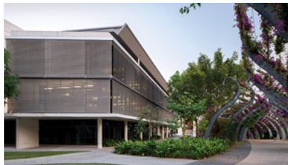
A layer of aluminium operable screens filters light for the interiors and multiple workstations.
