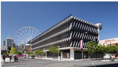
Steel blades ripple across the ABC building's northern and western facades.
