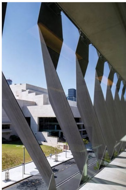
Blades made from 10mm high-tensile grade 350 BlueScope steel plate deflect sound and double as sunscreens.
