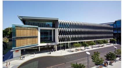
Broadcasting studios have a prime view of South Bank Parklands from the cantilevered glass boxes.
