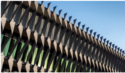
A striking pattern of steel blades give the new ABC Brisbane Accommodation building its striking exterior identity.
