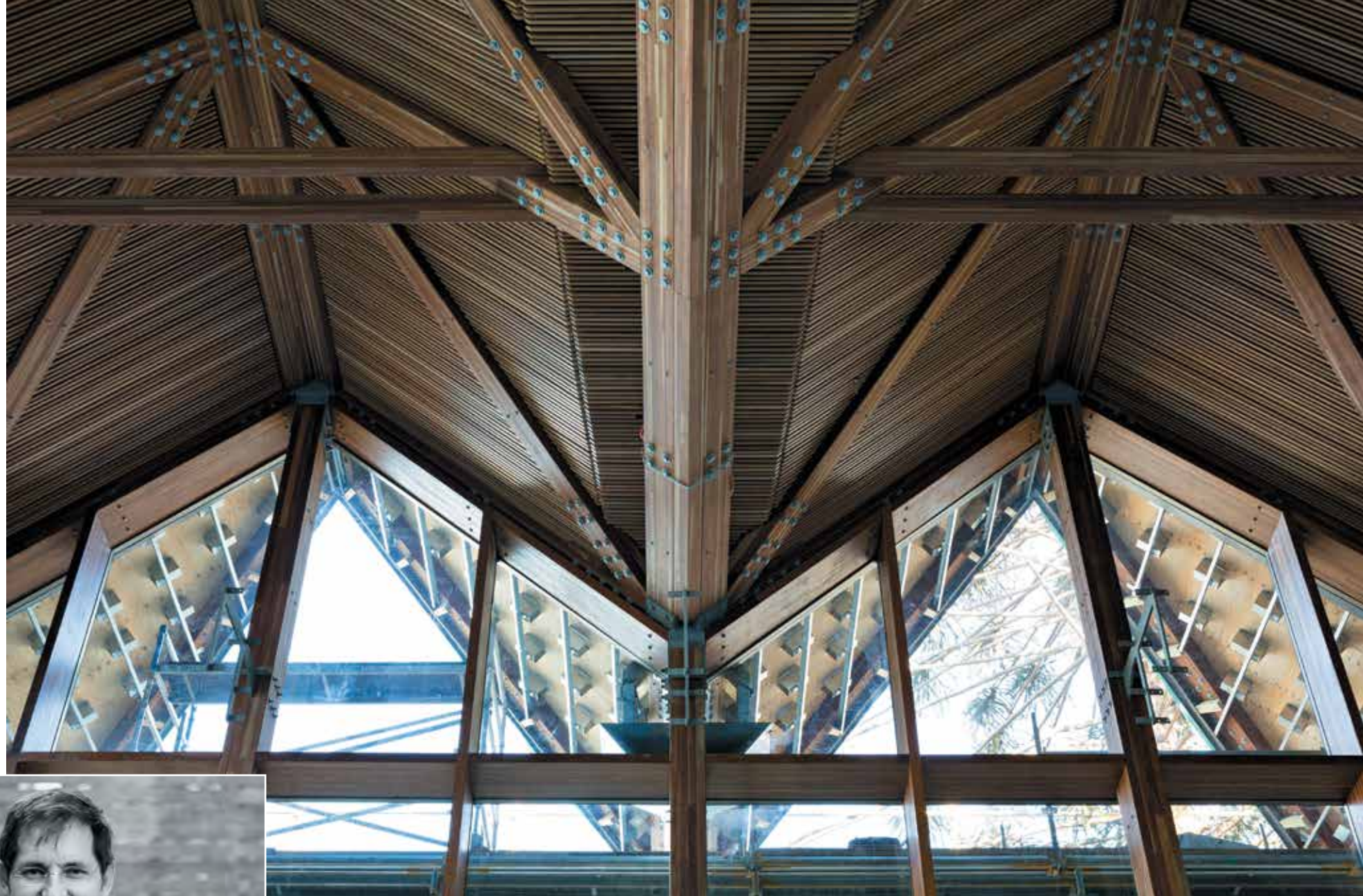
To express the auditorium externally and achieve greater structural capacity, the roof was formed as a series of folded plates
