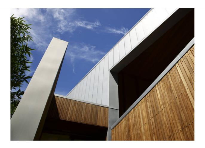
The northern face of the building form is articulated by rotating the external walls 15 degrees. The walls peel away from each other resulting in thin vertical fissures which allow northern light and breezes to filter through. The vertical fissures afford the significant rooms of the house a private visual connection to views down the longest reach of the Brisbane River.
