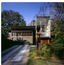
( http://www.contemporist.com/the-lockyer-residence-by-shaun-lockyer-architects-with-arkhefield/ ) The Lockyer Residence by Shaun Lockyer Architects with Arkhefield
