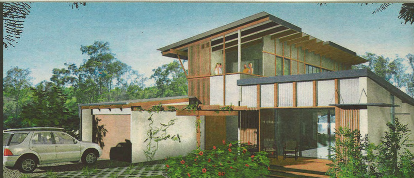
Driftwood will have designs from various architects at Dicky Beach, above ; Malcolm Middleton-designed house at Seaspray, inset below
